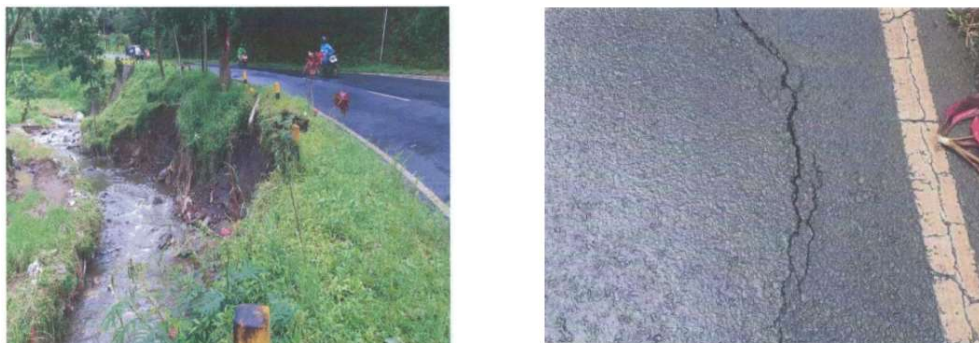
Figure 2. Photos of Early Avalanches and Early Cracks
