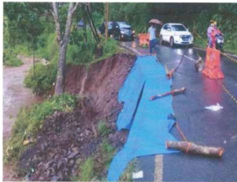
Figure 3. Avalanche to the edge of the pavement
