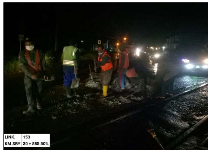
Figure 2. Repair with CTB and HRS at JPL 67
