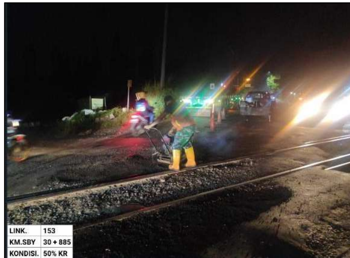
Figure 5. Cold Mixed Overlay at JPL 67
