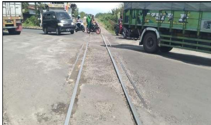
Figure 6. Cold Mixed Asphalt Overlaying Results
