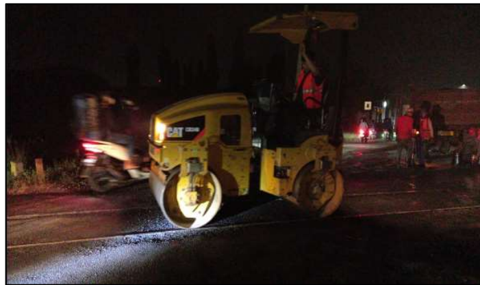
Figure 8. Repair with CTB and HRS at JPL 67
