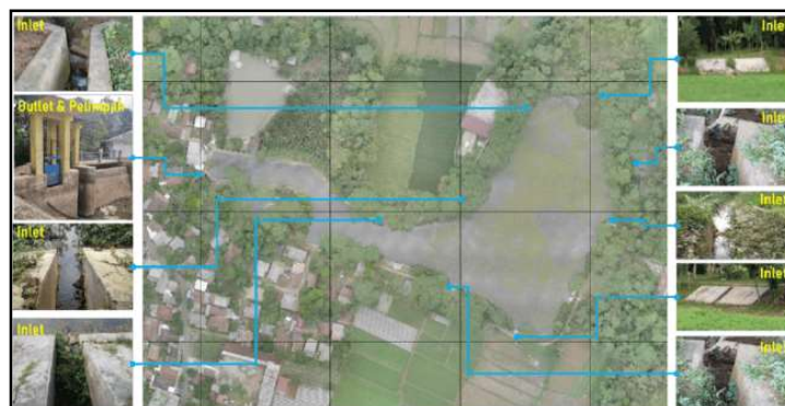
Figure 2. Existing Condition of Situ Kadupayung Source: Consultant Survey Results, 2023
