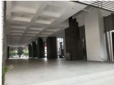
Figure 5. Open space on the ground floor
