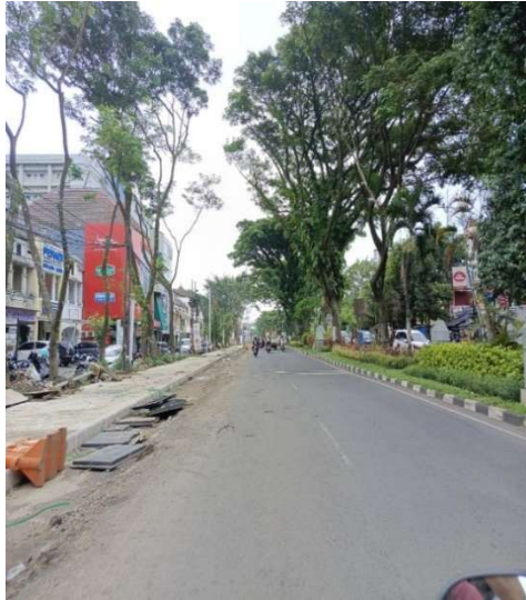
Figure 5. Condition of the Jalan Soekarno Hatta Street Sidewalk Source: Results of data analysis, 2025
