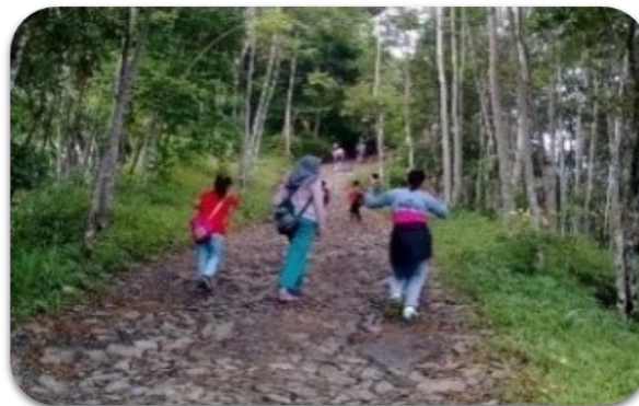
Figure 3. Condition of the Pamalayan village road in Cisewu District Source: Researcher documentation, 2025
