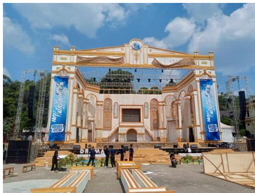
Figure 2. Stage Installation Process, Source: Darul Amanah Documentation
