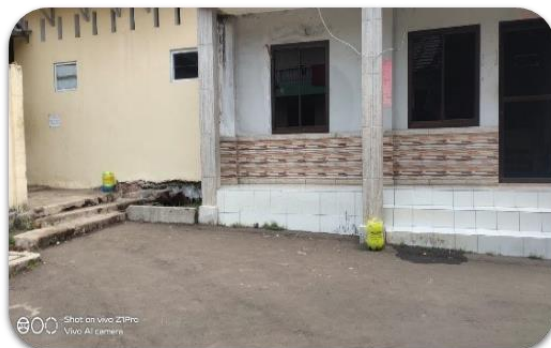
Picture 2. Placing trash bins at designated points and creating trash bins
