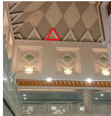
Figure 3. Ceiling of the Sheikh Yusuf Gowa Grand Mosque
