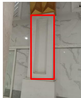
Figure 7. Wall of the Sheikh Yusuf Gowa Grand Mosque
